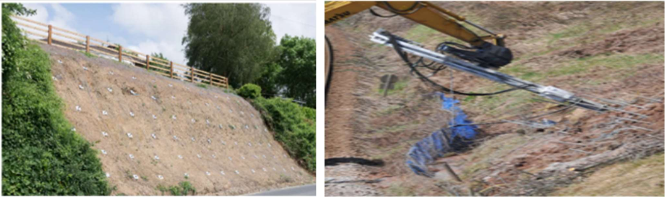
Figure 5-130 Example of Soil Nail Installation
