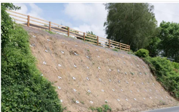
Figure 5-6 Typical Soil Nail / Anchor Installation
