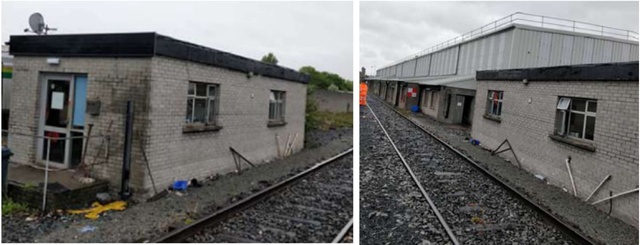
Figure 5-68 Shunter Building to be Removed
