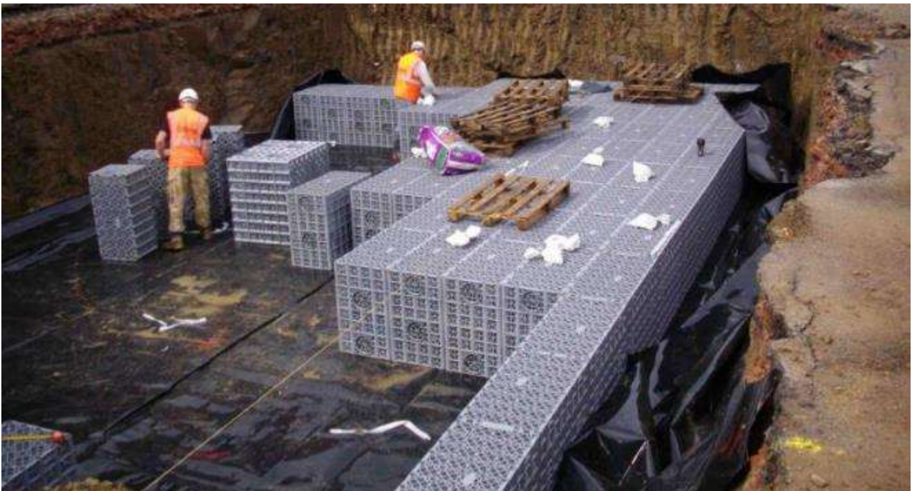
Figure 5-8 Typical Modular Attenuation Tank
