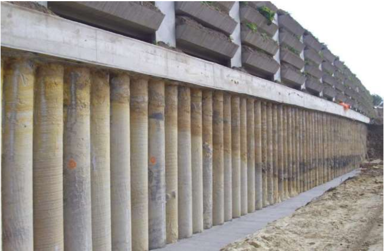
Figure 5-2 Example of a Bored Pile Wall
